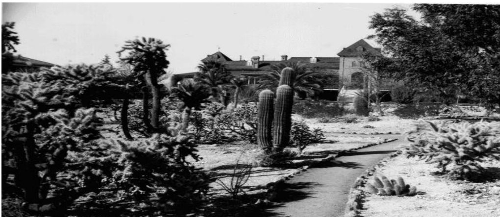
1893 Old Main At University Of Arizona
